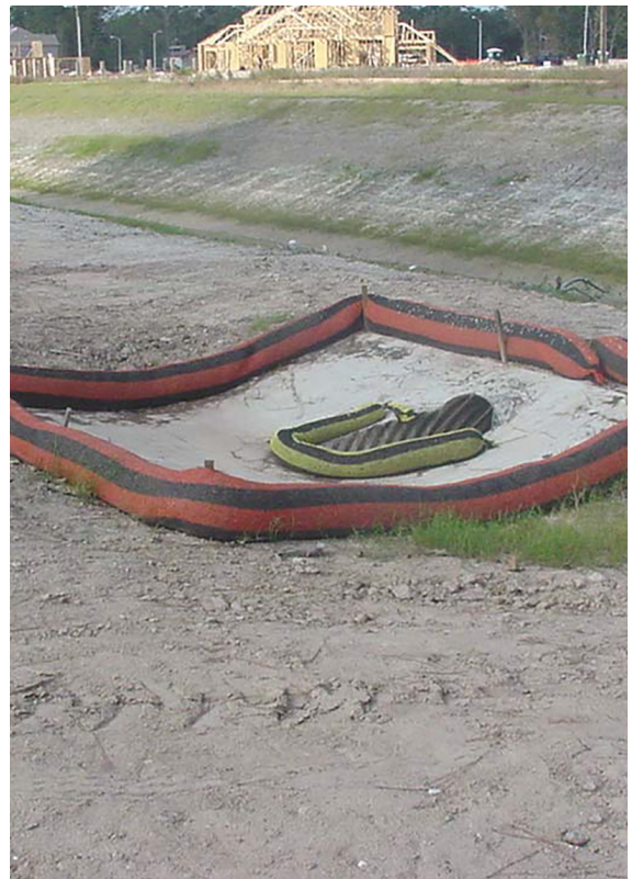
Compost filter sock protects an inlet drain.
