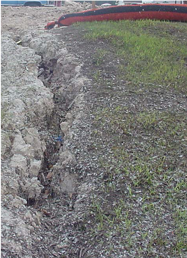
Comparison between hydro mulch on the left and a compost filter sock on the right.
