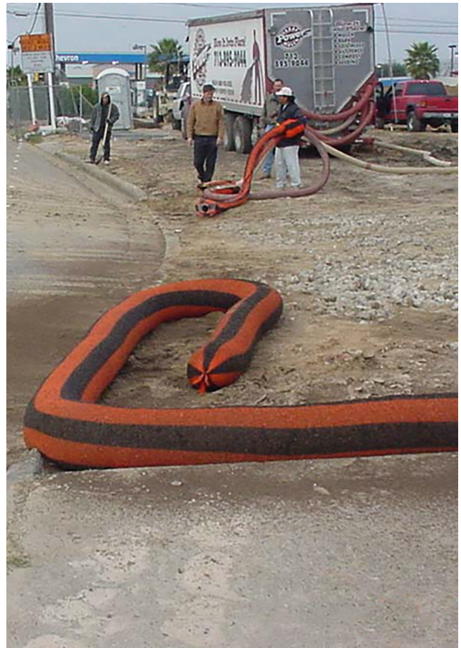
Compost filter sock being used as a gate to halt erosive flows. Photo Credit: Texas Commission on Environmental Quality and the Texas Department of Transportation
