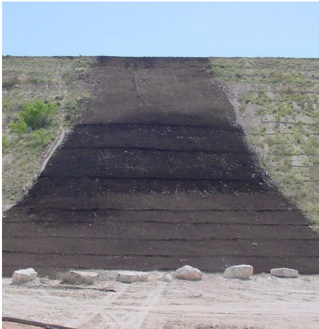
Compost blanket in conjunction with multiple filter berms. Photo Credit: Texas Commission on Environmental Quality and the Texas Department of Transportation
