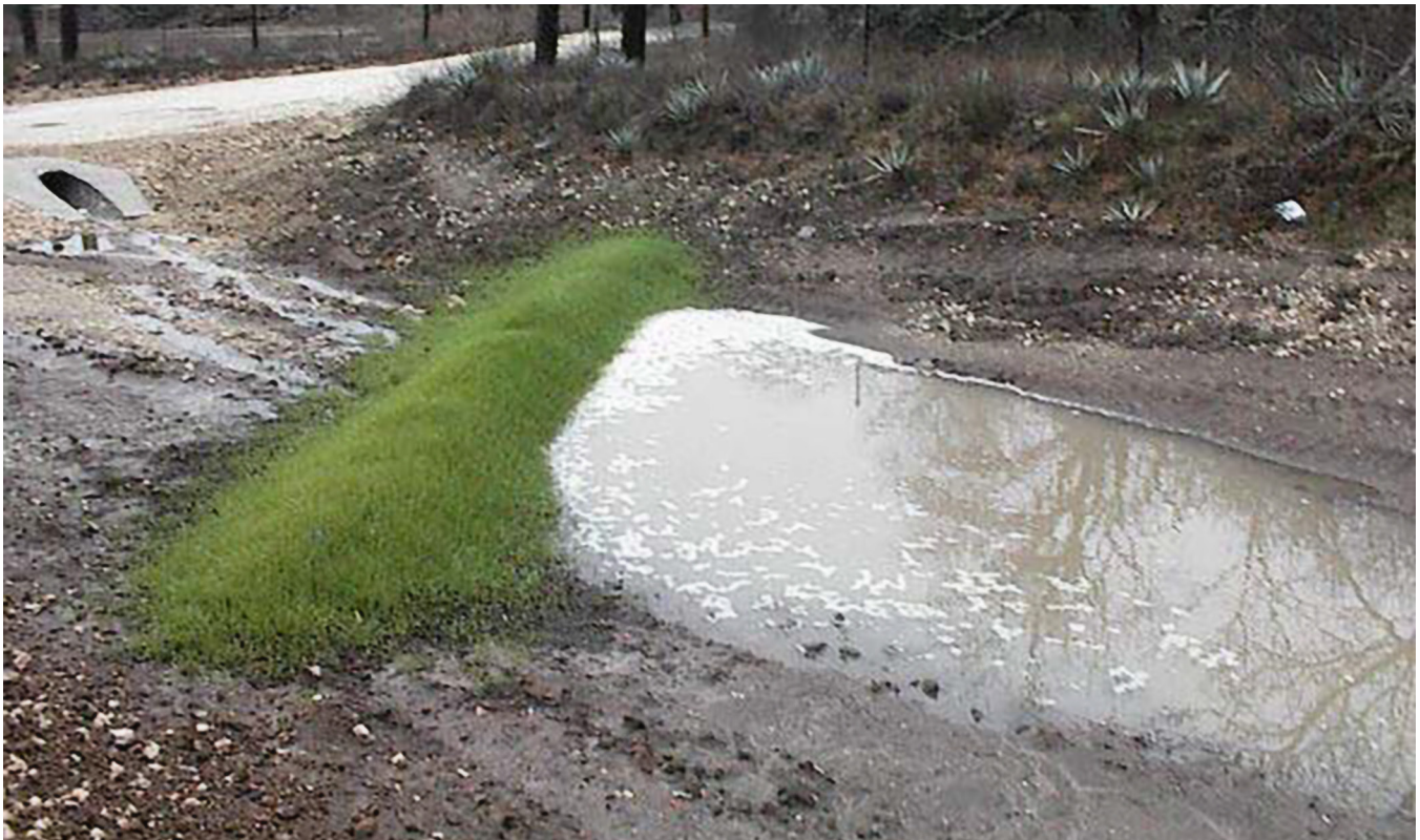
Filter berm working during a rain event.
