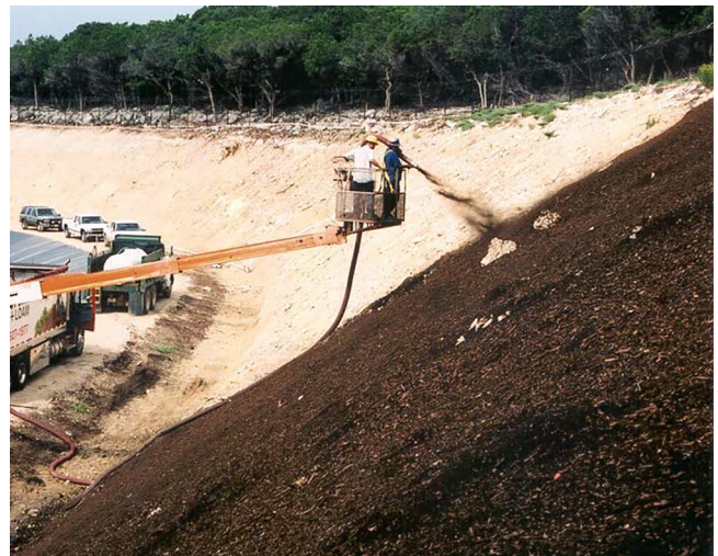
Application of seeded compost blanket on a 1:1 Rock Slope Photo Credit: Texas Commission on Environmental Quality and the Texas Department of Transportation
